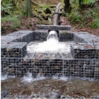
Evans Creek HDPE pipe outfall energy dissipation
