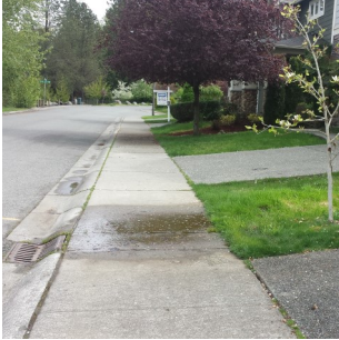
Example of groundwater seepage
