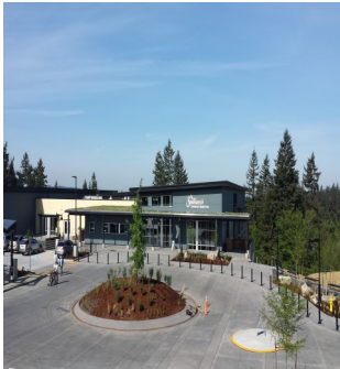
Sammamish Community and Aquatic Center green roof
