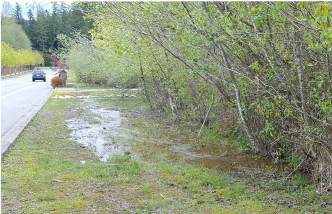
FIGURE 7. FLOODED DITCH ADJACENT TO 248 TH AVE SE.
